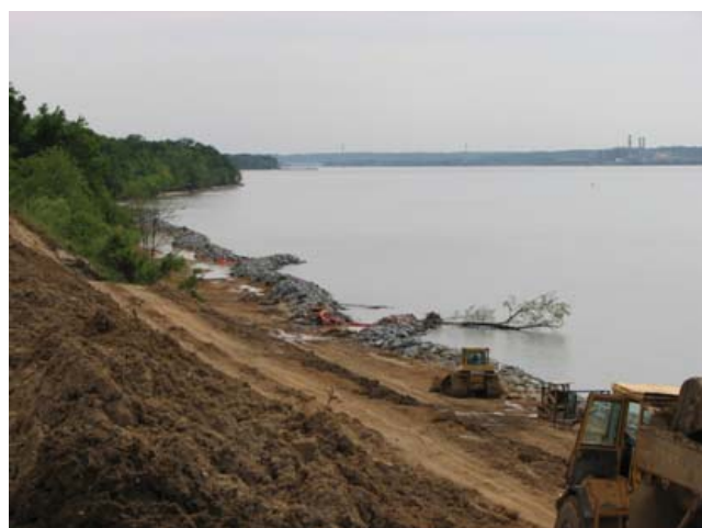
Slope and sill grading that took place in 2008.
