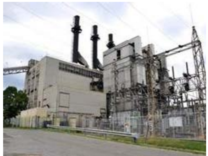
Photo courtesy of the U.S. NAVY Goddard Power Plant, the last coal-fired power facility operated by the Navy, will be demolished and replaced in a $62.45 million military construction project on Naval Support Facility Indian Head that gets underway this month. The project will decommission the Goddard plant, built in 1957 and now well past its operational life span and unable to meet current emission standards.
