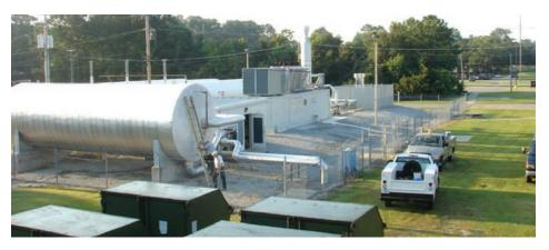
An ESPC was used to install a 1 MW cogeneration plant that supplies heat to the barracks, mess hall, and medical facility. *Photo from U.S. Marine Corps Air Station Beaufort*
