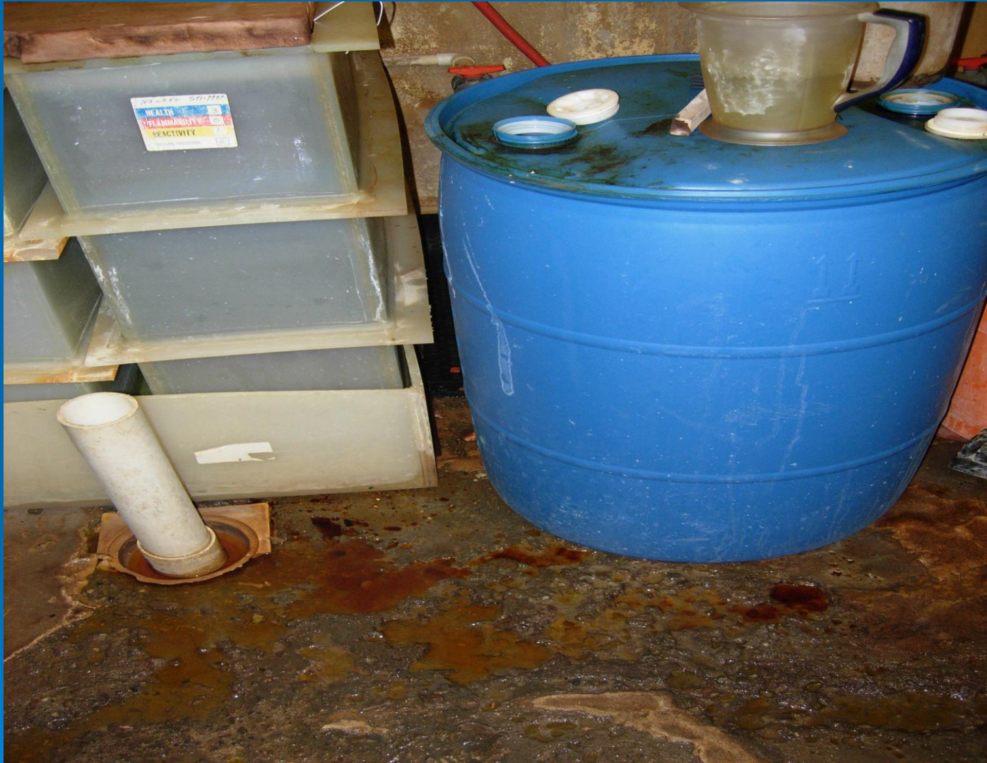
Floor drain in a chemical storage area
