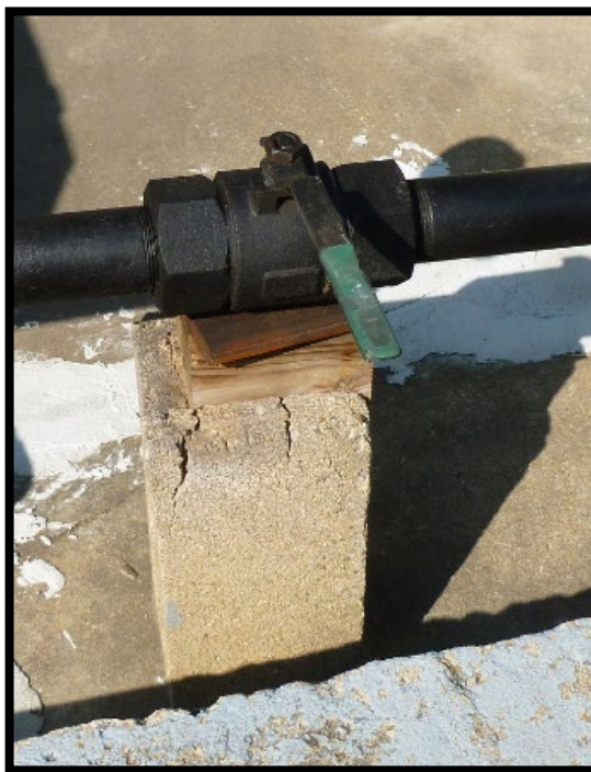
Piping Supports not Proper
