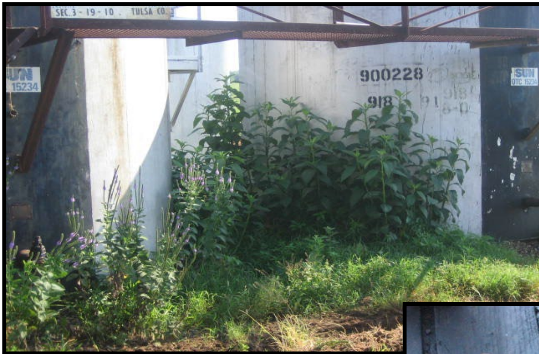
Excessive Vegetation Growth in Containment Area
