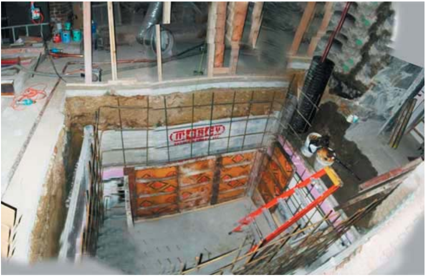
Construction of an elevator pit
