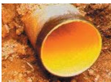
Left: A digital subsurface image during an inspection. Right: A completed, cured in place, repaired pipe
