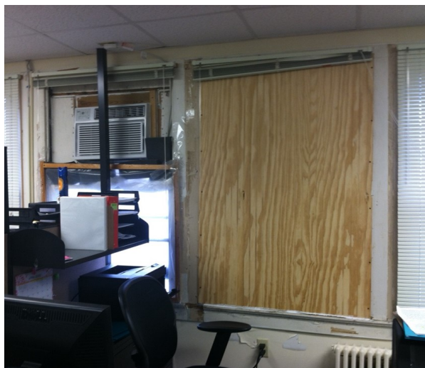
Above: Inside view of leaking windows in Building 409.
