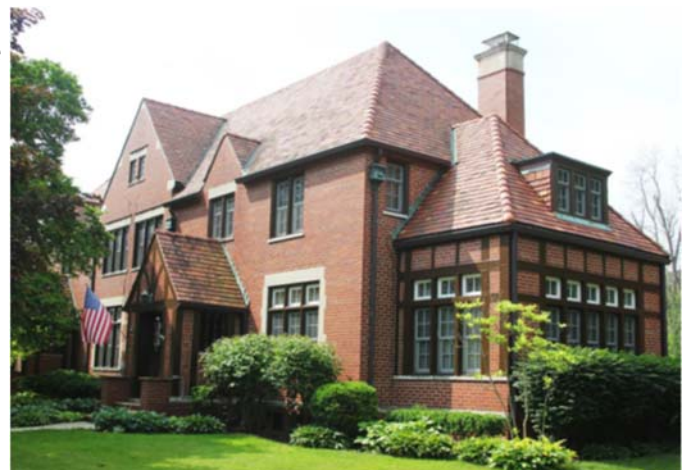
Above: The Air Force is working closely with the Ohio SHPO and the ACHP to explore alternatives, including an innovative look at NHPA Sec. 111 out-leasing, to ensure preservation and continued use of Wright-Patterson AFB's WWII era Brick Quarters housing ( http://wpafbhousingeis.versar.com/ ).
