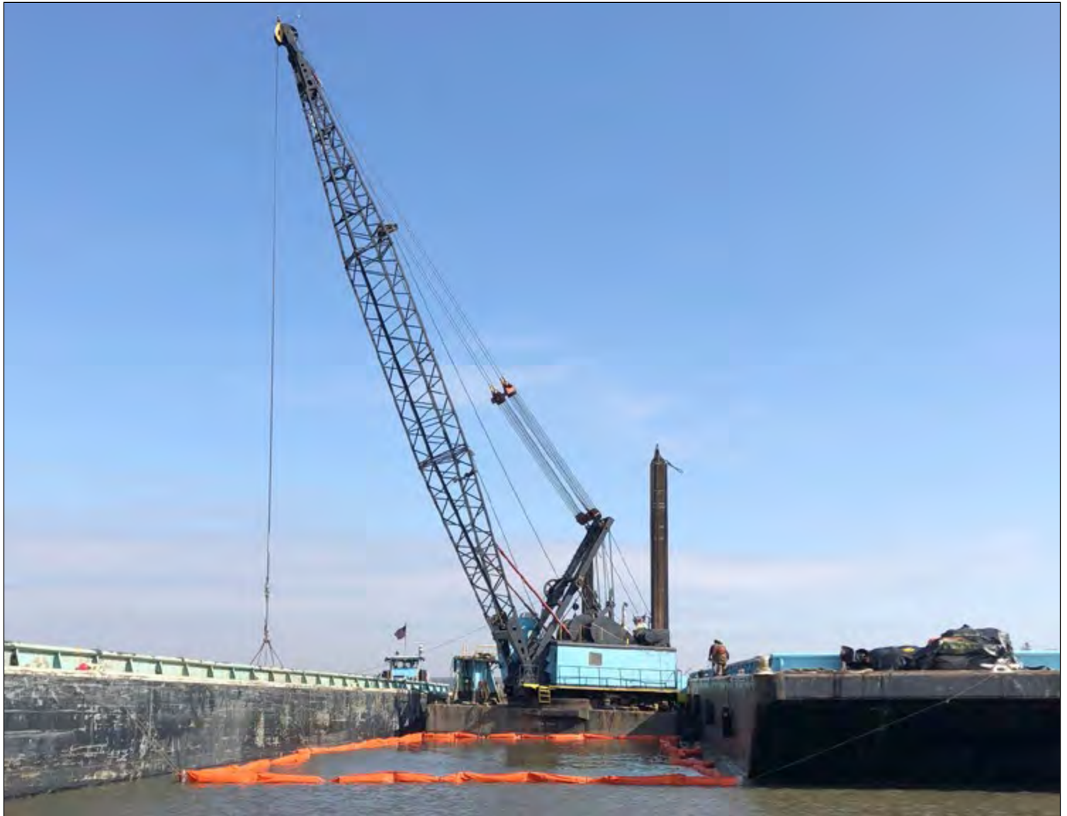
A dredge excavates material from the North Cove Federal Navigation project in Old Saybrook, Connecticut.
