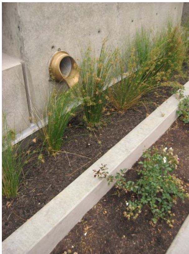
Figure 9. Disconnected downspout discharging to planter box.
