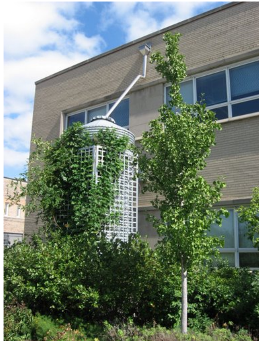
Figure 5. Rain water cistern.
